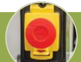
EMERGENCY POWER OFF SWITCH
